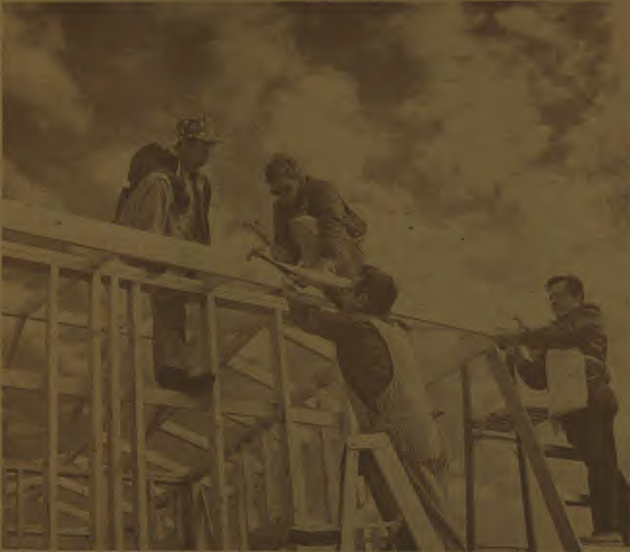
SEVERAL kinds of framing construction are represented in this storage shed being built by apprentice carpenters. Instructor Frank Lesperance, left, gives the word to Jerry Smith, Al Ayott and Milton George (all 7513). The Plant Technician apprenticeship program requires 10,000 hours of classroom and field training.
